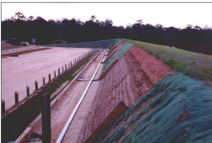
Figure 3-7. Fort Rucker berm and backstop.
