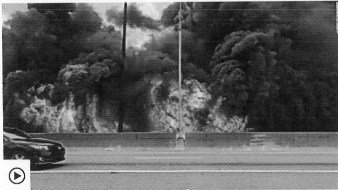
Inside Atlanta's 40-foot wall of fire
