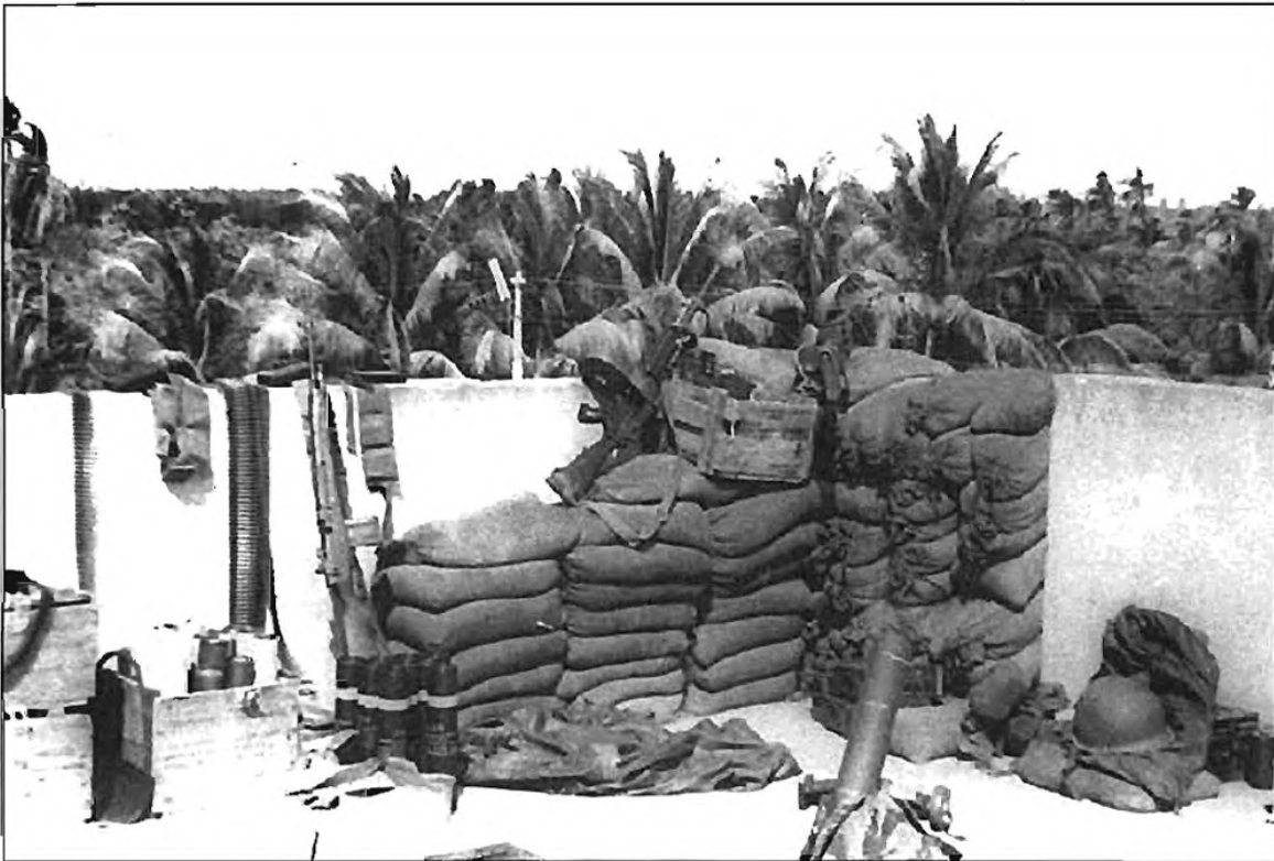
The fortifications put in place on top of a SEAL billet in Vietnam during the Tet Offensive of 1968. At the lower right of the photo can be seen an M1 steel helmet laying on top of an M69 armor vest. Next to the vest is a set of web gear including at least one canteen. On top of the sandbags can be seen the buttplate of a loaded M60 machine gun. Next to the M60, leaning against the crate of ammunition, is a Stoner 63A light machine gun with a 150 round belt drum in place for use. Leaning against the wall just to the left of the sandbags is an M14 rifle with a 20 round magazine locked into place. The bandoleers appear to be additional 7.62mm ammunition in stripper clips for the M14 and additional M14 magazine are laying on top of the wall. Belts of 7.62mm ammunition for the M60 and 5.56mm belts for the Stoner are both draped over the wall. At the base of the M14 are the black fiberboard tubes holding high explosive ammunition for the M29 81mm mortar, the top portion of which can be seen just to the right of the center foreground of the picture.
